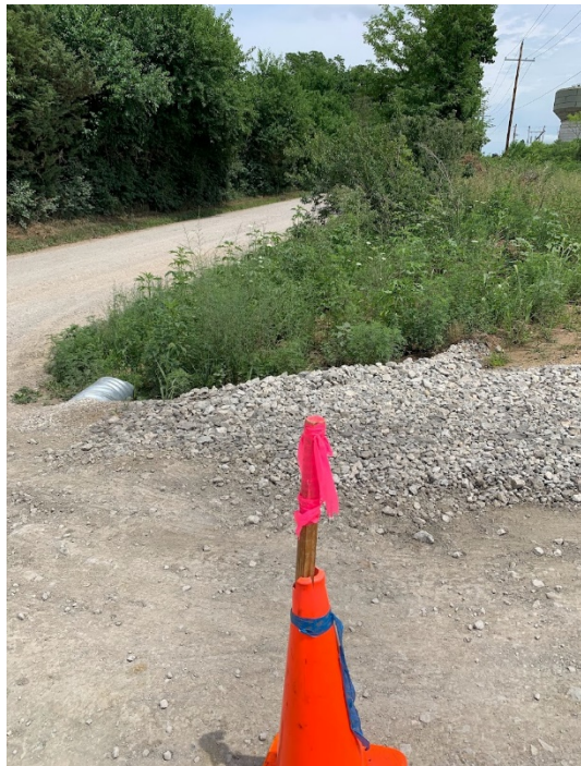
Kansas Avenue looking east at construction access
