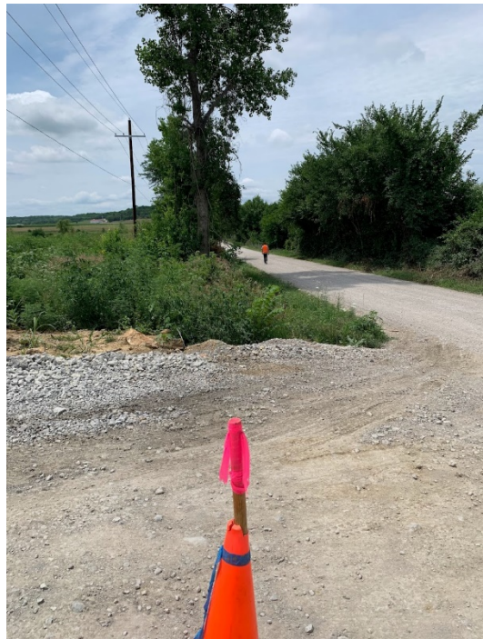
Kansas Avenue looking west at construction access
